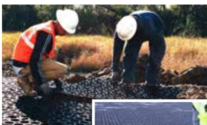
Place TRUEGRID PRO PLUS and connect.
