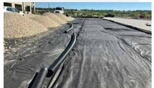
Install under drain system, if specified.
