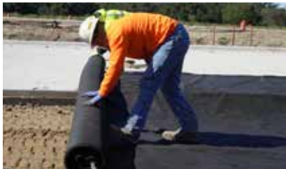
Place Geotextile fabric and pin overlaps.
