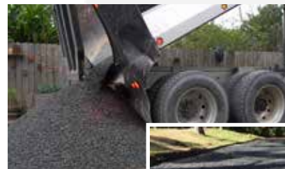
Place and spread fill material.
