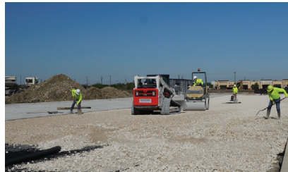
Place and compact base material. Compact in 4" Lifts.
