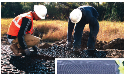
Place TRUEGRID PRO PLUS and connect.
