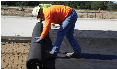
Place Geotextile fabric and pin overlaps.
