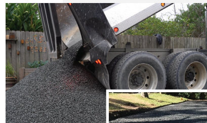
Place and spread fill material.
