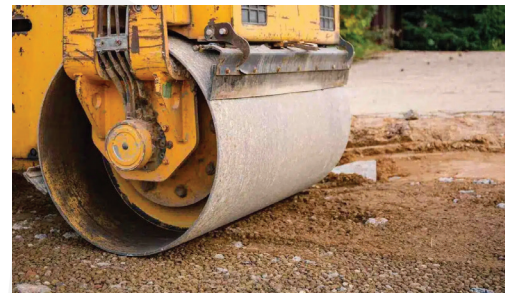
Compact subgrade with rolling compactor or other equipment.
