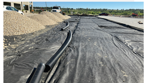
Install under drain system, if specified.
