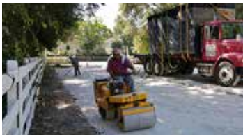
Place and compact base material. Compact in 4" Lifts.
