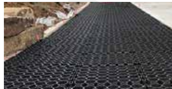
Place TRUEGRID PRO PLUS and connect. Cut as needed.
