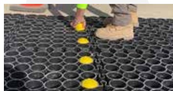
Place SuperSpots, SnowSpots™, and Plates™ prior to filling TRUEGRID.
