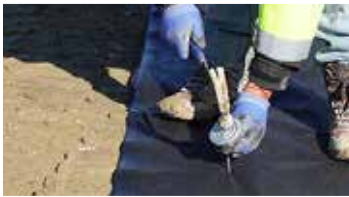
Place Geotextile fabric and pin overlaps.
