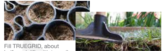
Use rolling, plate, or hand compactor to compress sod into cells.
