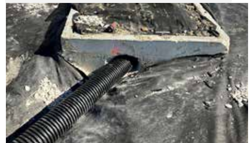
Install under drain system, if specified.
