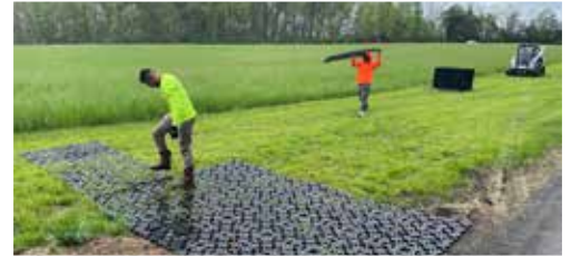
Line-up ROOT pieces with receiver tabs facing out. Connect to the next piece or sheet with empty cells facing down and grid-side up.
