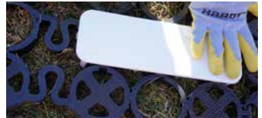
Position and insert ROOT STRIPES, if included on project, prior to compaction.
