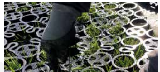
Use sod staples or other pins, as needed, on edges or and other areas to secure ROOT.
