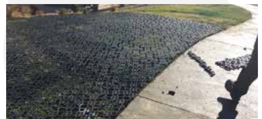
Cut to fit the area to allow for sprinkler heads, curbing, or other obstacles. Mechanical saws are recommended.
