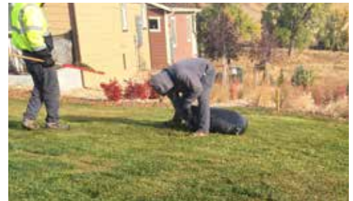
Level out any ruts, and remove any debris from the surface.
